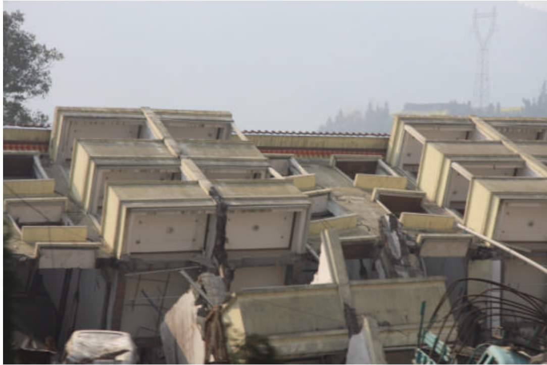
Buildings were completely destroyed in Yingxiu County, very close to the epicenter.
