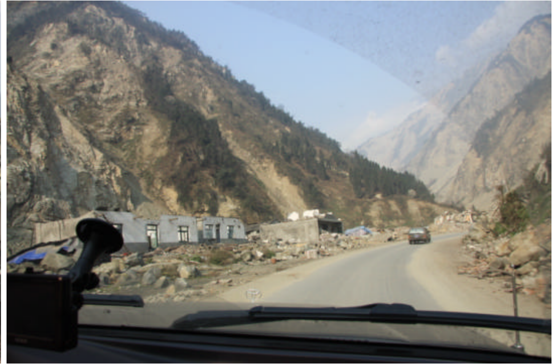
Houses along the way to Wolong Nature Reserve completely collapsed.
