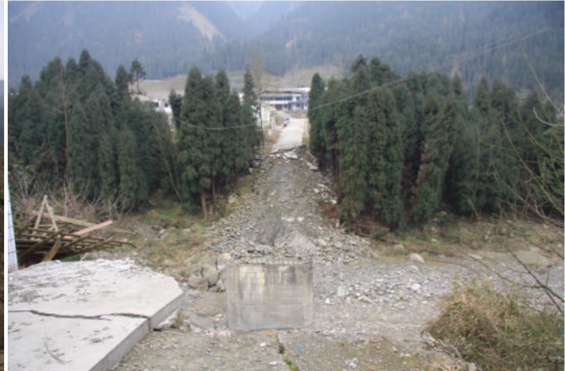
Wangjiaping station, a communications and education center, and its front bridge were destroyed. The rangers were right there when earthquake happening, but nobody dead. They got out to rescue the local villagers.
