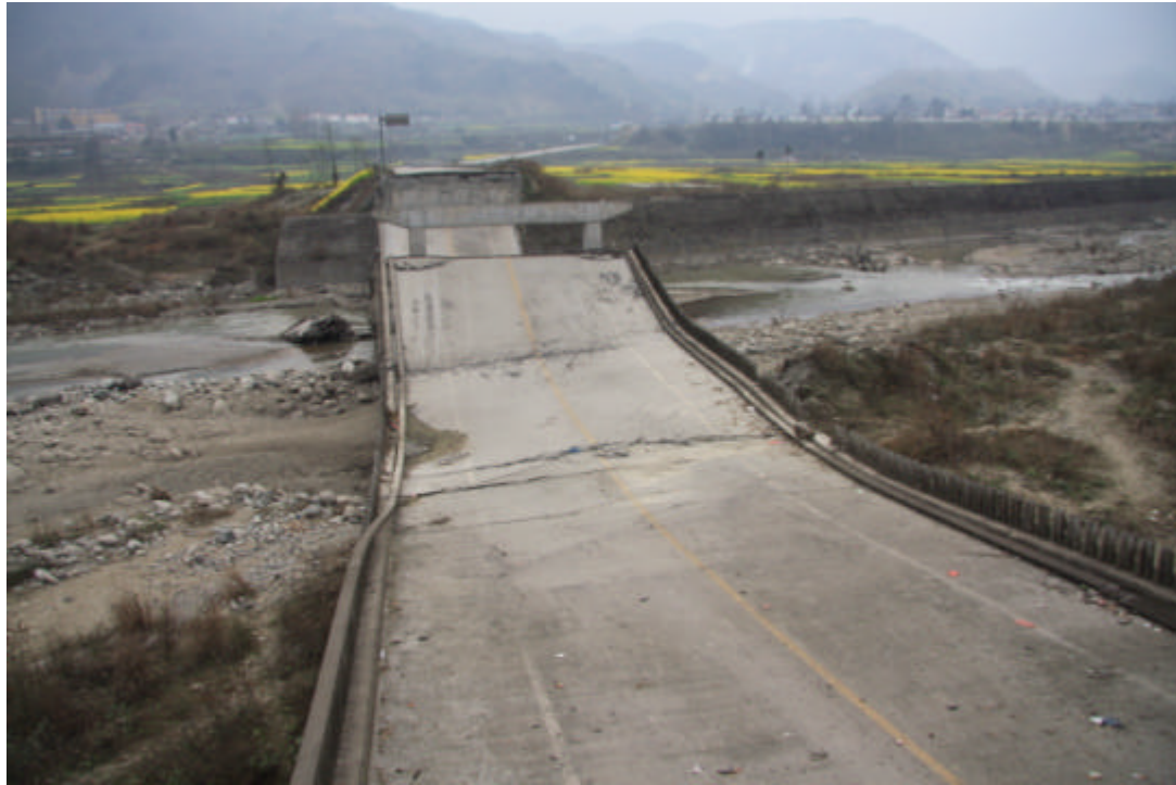
The Xiaoyudong bridge, one of memorial scene with yellow flowers along riverbeds to Baishuihe Nature Reserve, was collapsed.
