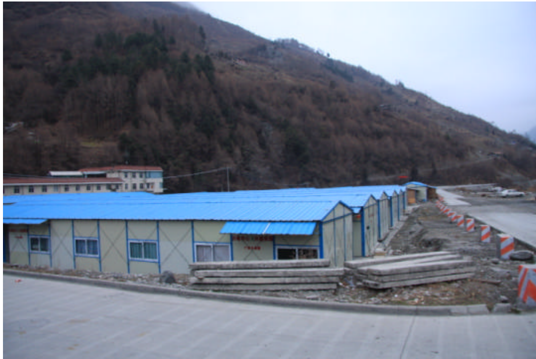
Administration bureau buildings in Wolong Nature Reserve were destroyed and all closed for reconstruction. Local governments, administration bureau and villagers use the temporary shelters for living and office affairs.
