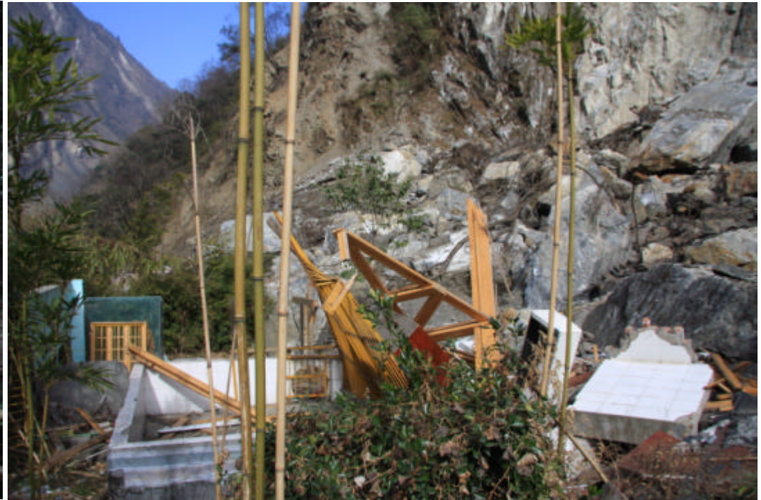
All facilities in the Center were totally destroyed.
