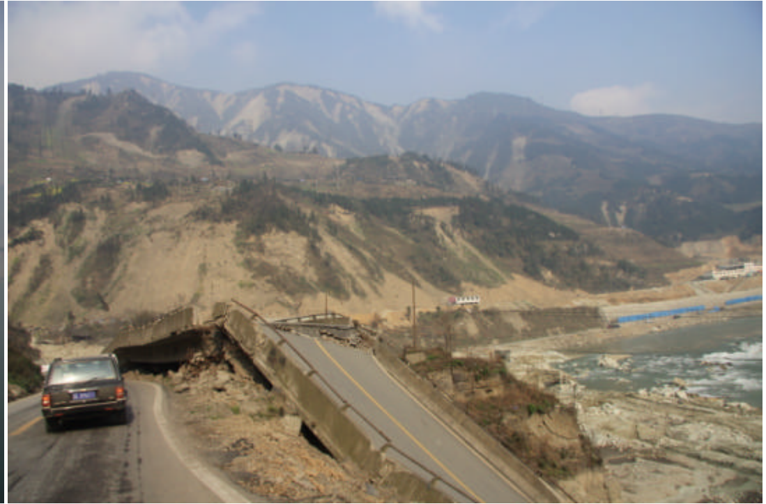
Besides the severe causes of landslides, infrastructures of roads, bridges, tunnels, and dams were also severely damaged along the way to Wolong Nature Reserve.
