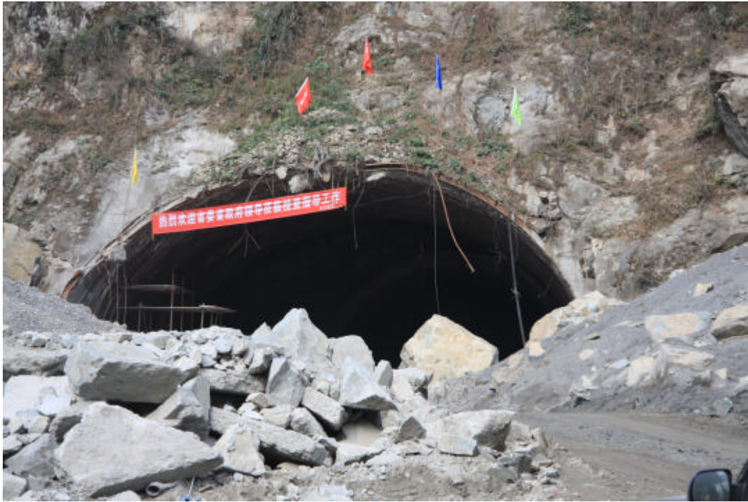
Tunnels to the Wolong Nature Reserve were buried.
